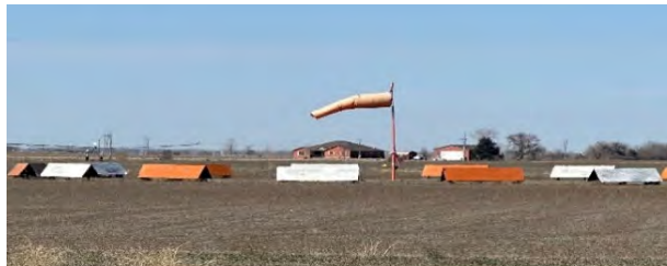
Lighted Wind Cone and Segmented Circle
