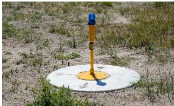
Example Taxiway Edge Lighting Fixture
